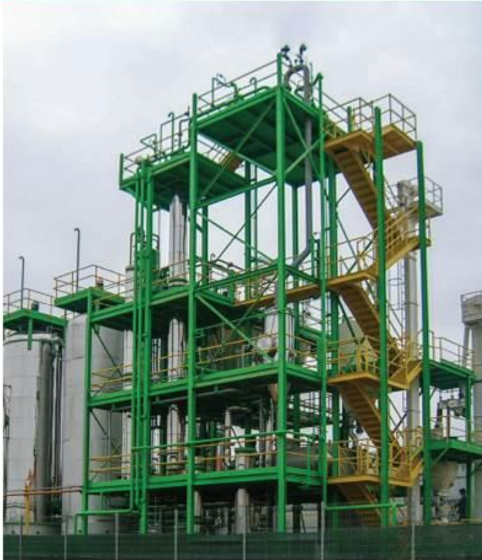
PERSEO Bioethanol® Pilot Plant
